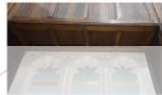
Soffit- Photo Ref*
